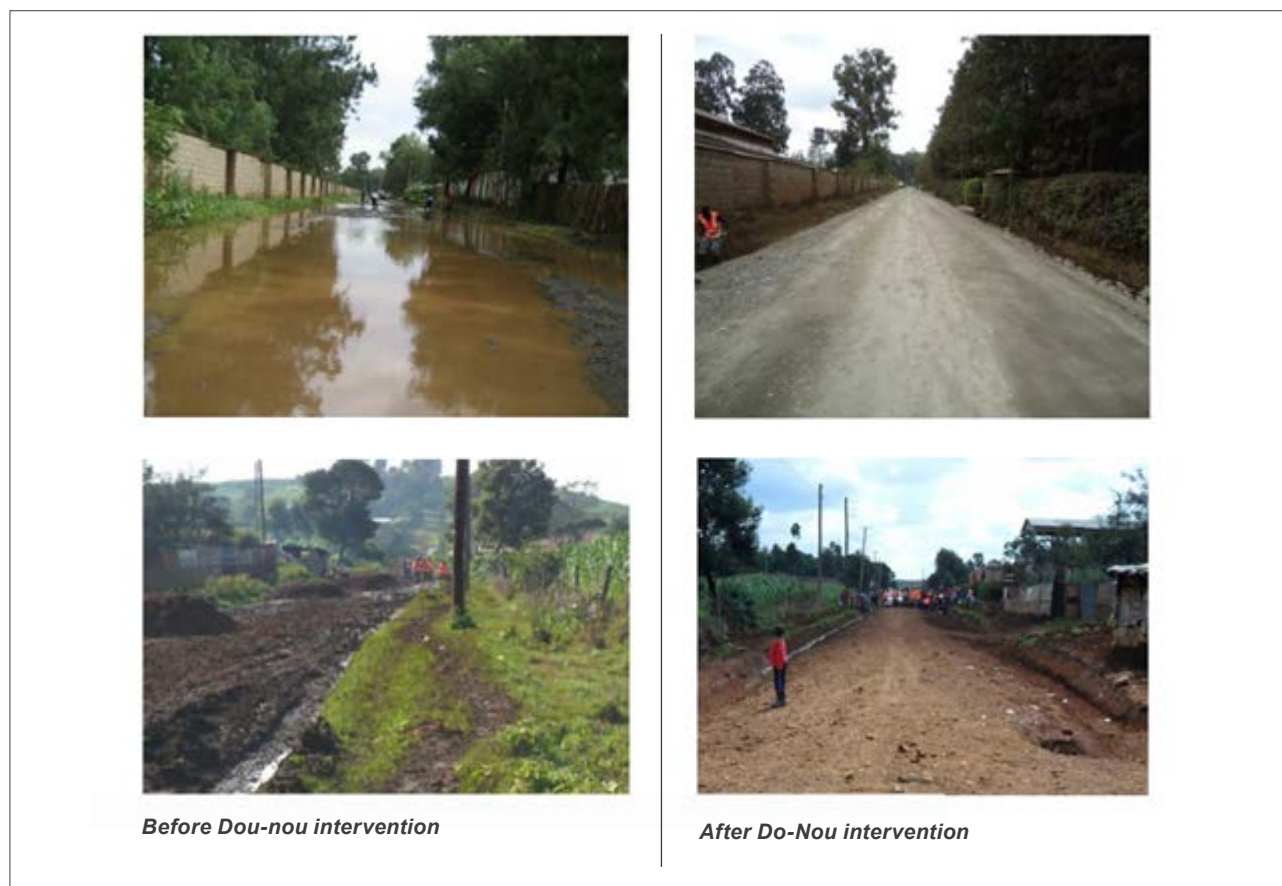
Figure 14.6 Illustration of Application of Do-Nou Technology to Waterlogged Road Section
